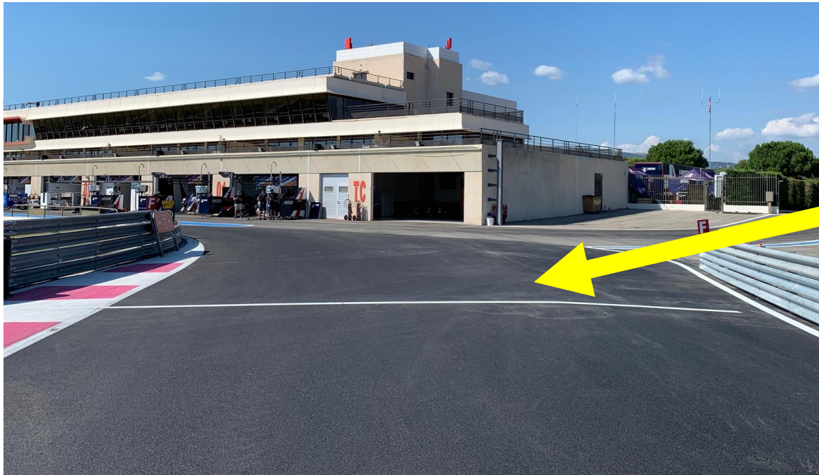
START OF THE WORKING AREA
